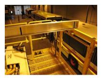
5) Set beam on top of handrail. Black marks on "I" beam indicate position for clamping. Two positions allow for hoist to travel off either one side or the other to lower module to ground.
