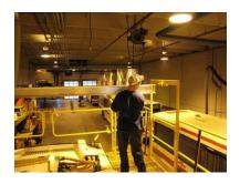
7) Slide beam in one end and then shift beam opposite way to support both ends. Black marks on "I" beam to be centered under support point.
