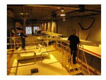
4) Together move beam into place from platform to platform.
